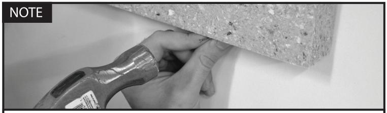
We recommend using finishing nails in the wall at bottom of the tiles to help to support while the adhesive cures. Preventing the Tile from sliding.
