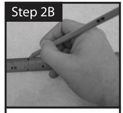
For isolé make two level marks 16" from either side of center mark.
