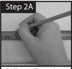
For Absorption Sheets make two level marks 23 3/4" from either side of center mark.
