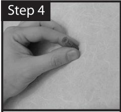
For drywall we recommend inserting anchors into pre-drilled holes.
