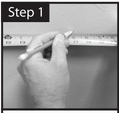
Start by measuring and marking center of intended hanging area.
