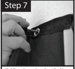
Holding absorption sheet/isolé up to the wall, line up grommet holes with predrilled holes and screw in your prefered hardware.
