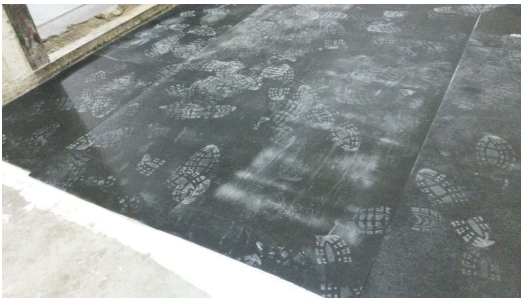
Figure 2 – Detail of underlayment prior to joint treatment
