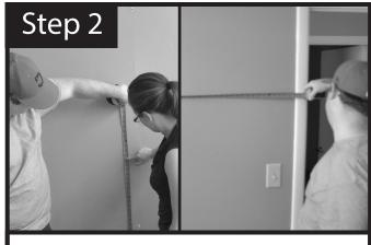
Measure installation wall to find appropriate placement for center panel based off of overall size of arrangement from step 1.
