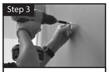
Place the top offset mounts for your center panel according to measurements from step 1.
