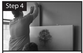
After Installing the center panel, start placing your additional panels around it and marking the Z-Clip placements.
